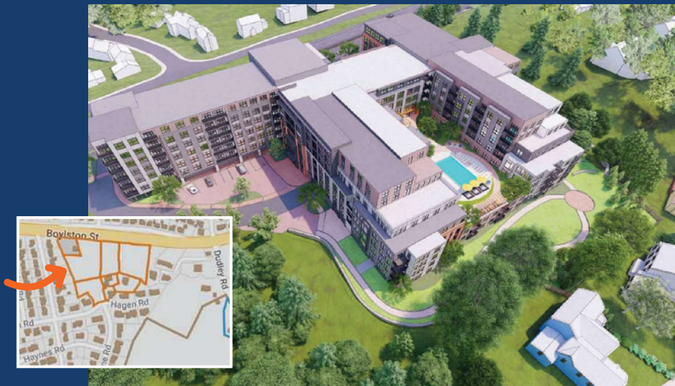
Location & Overhead View of 528 Boylston Street
